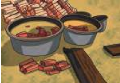
Figure 6.14: Bricks are soaked in water before use
