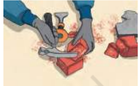
Figure 6.16: Cutting the brick using chisel and hammer
