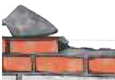
Figure 6.15: Applying mortar while laying bricks
