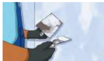
Figure 6.20: Plastering of a wall
