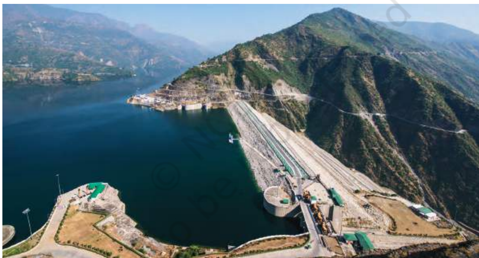
Figure 6.1: Tehri dam in Uttarakhand
