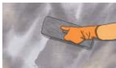
Figure 6.19: Applying plaster on the wall
